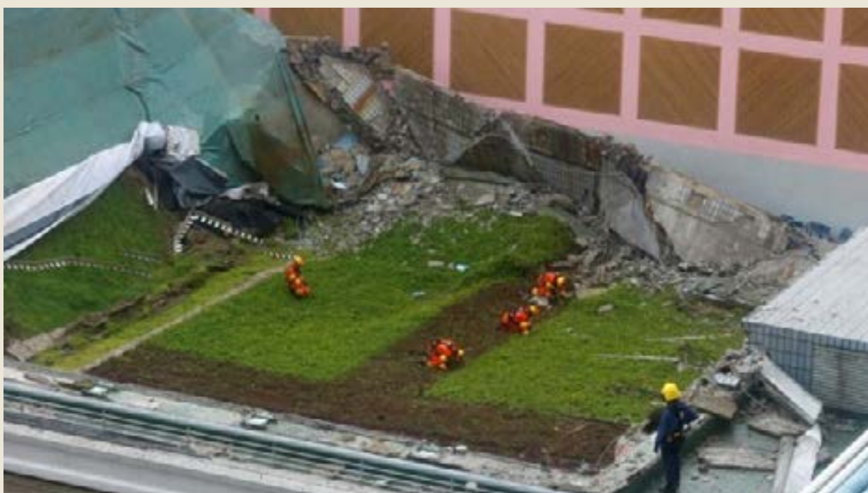
The roof had been covered with grass
